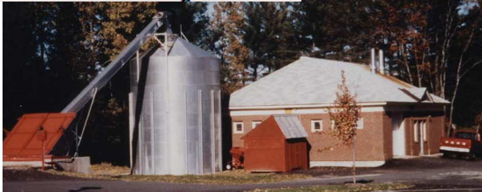
Lyndon Town School, Lyndon, Vermont System Size: 1.2 MMBH Manufacturer: Chiptec Wood Energy Systems This system uses an above-grade metal silo and separate boiler house (which includes garage space). Silo is loaded from a receiving bin (on far left) using an inclined auger.
