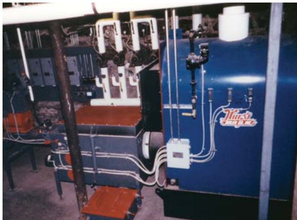
Shelburne Farms, Shelburne, Vermont Facility Type: Farm educational center System Size: 2.1 MMBH Manufacturer: Chiptec Wood Energy Systems
