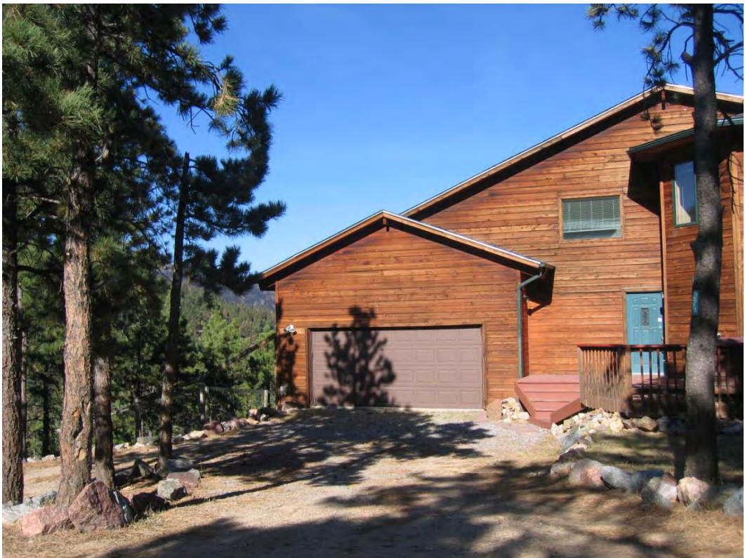
Figure 13. A total of 474 homes were located in the area where the Fourmile Canyon Fire burned. Photos: Russ Graham.
